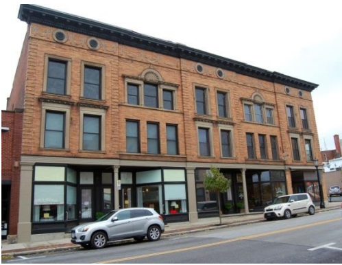
The Loft, 25 South Washington St.
